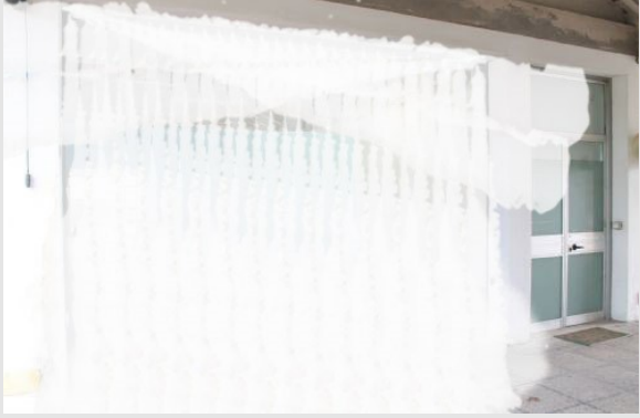
Barrier with water mist blade Spraytecs installed in a compartment of access to industrial warehouse.
